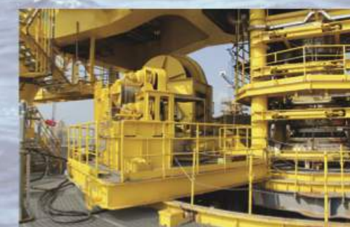
200 ton Riser Pull-in Winch System for ASENG FPSO
